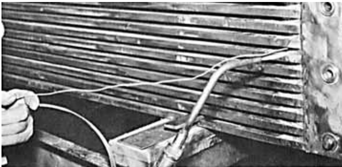
FIG. 28 Brazing repair
